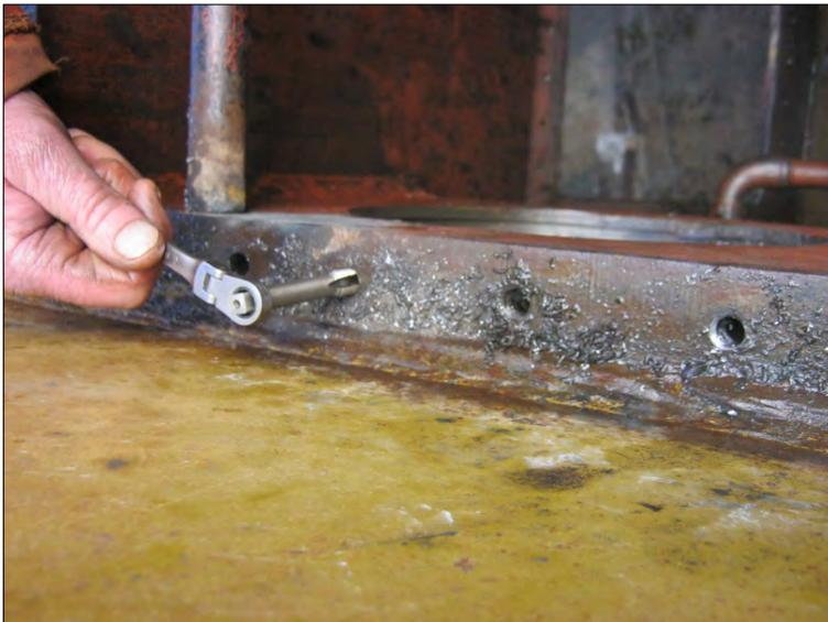
Re-tapping toggle cover plate holes to ensure the cover plate is sealed
