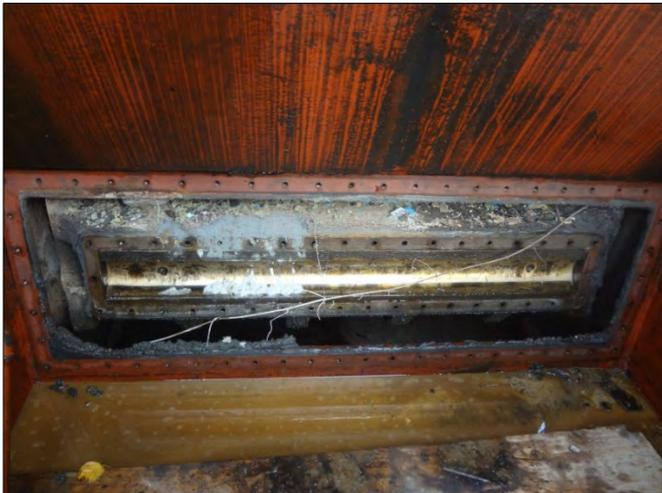
Removal of diaphragm and diaphragm frame.
