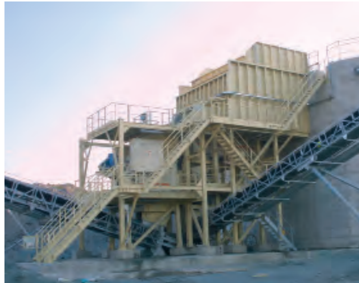
A C125 during the installation phase at a new primary crushing plant.
