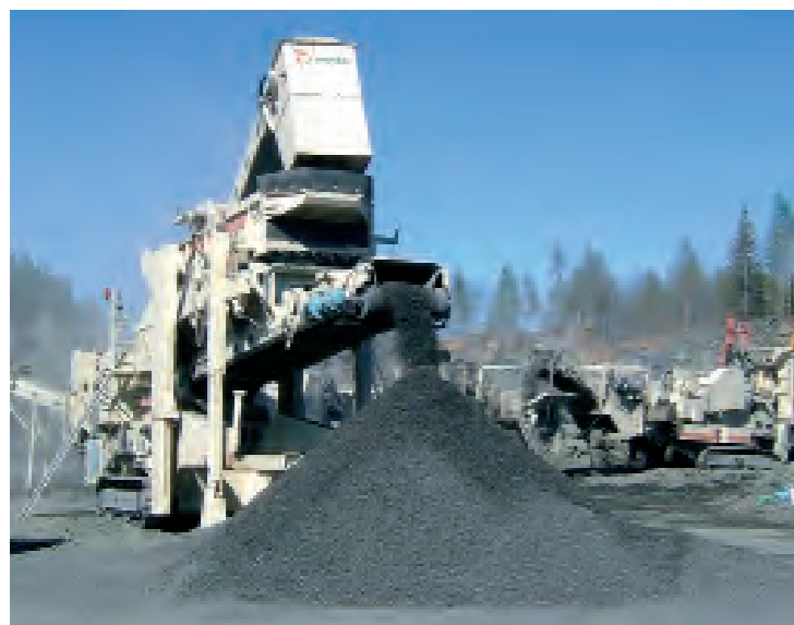
Three stage crushing and screening process with the Lokotrack LT110, LT300GP and LT300GPB.
